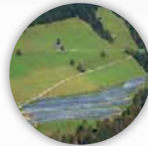
AUSTRIA - Small Power Plant 400kW
