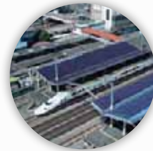
JAPAN - Platform 200kW
