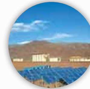
CHINA - Small Power Plant 30kW
